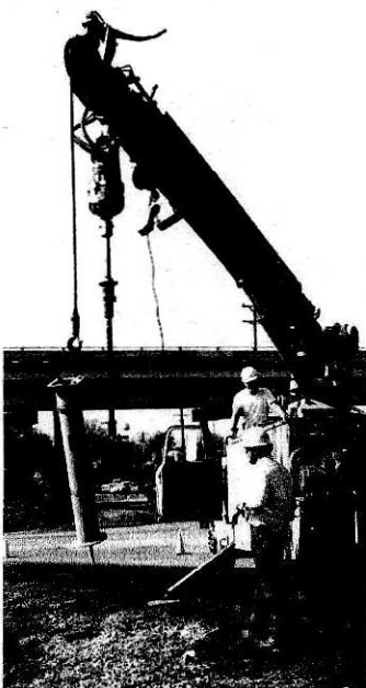
Unloading foundation from digger/derrick truck.
